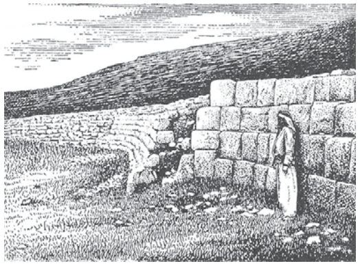
Assyrian Dam of rough masonry and mortared rubble, curved to withstand the flow of the river Khosr, Nineveh. Source: Singer, 1954.
